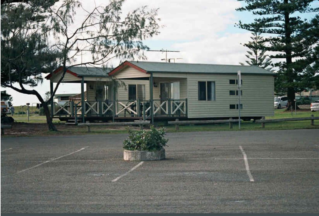
Cabins at Crescent Head – no attention to landscaping, unimaginative siting, no consideration of the interface between day-use and tourist accommodation.
