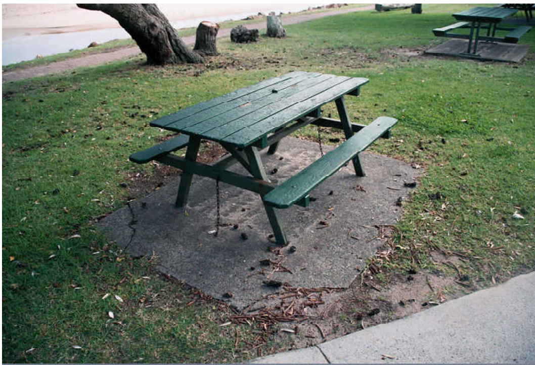
Crescent Head day-use facilities – outdated park furniture, poor maintenance, stumps not correctly removed.
